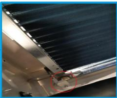
The resistance is activated when the external temperature is < 5°C
