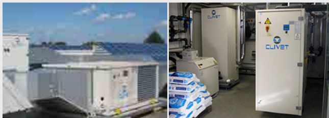
Conè – ZEPHIR dedicated outdoor air system with thermodynamic heat recovery and water-to-water heat pumps in the technical room
